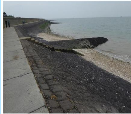
Open Stone Asphalt laid in 2005 at Two Tree Island
