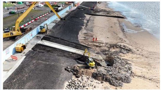
Placement of OSA/LSA at The Labworth
